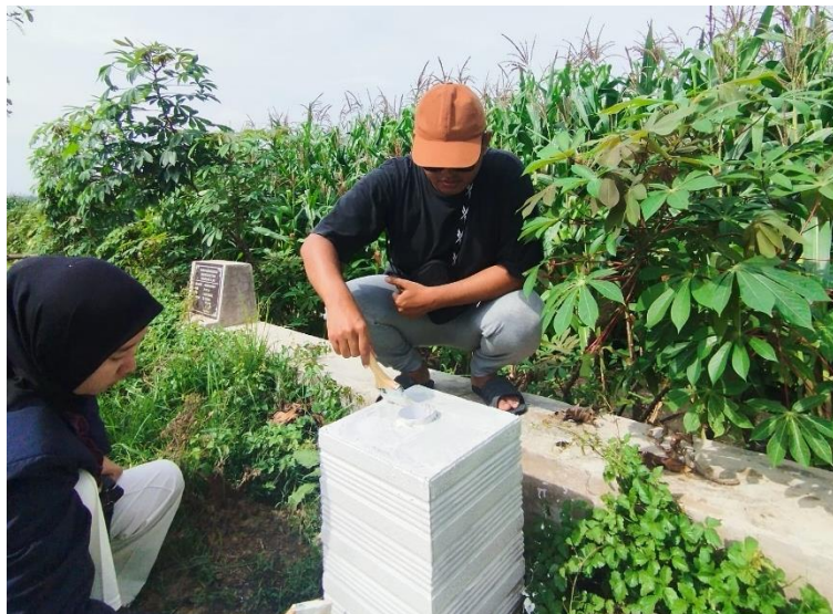
Gambar 2. Pengecatan umpak lampu panel surya
